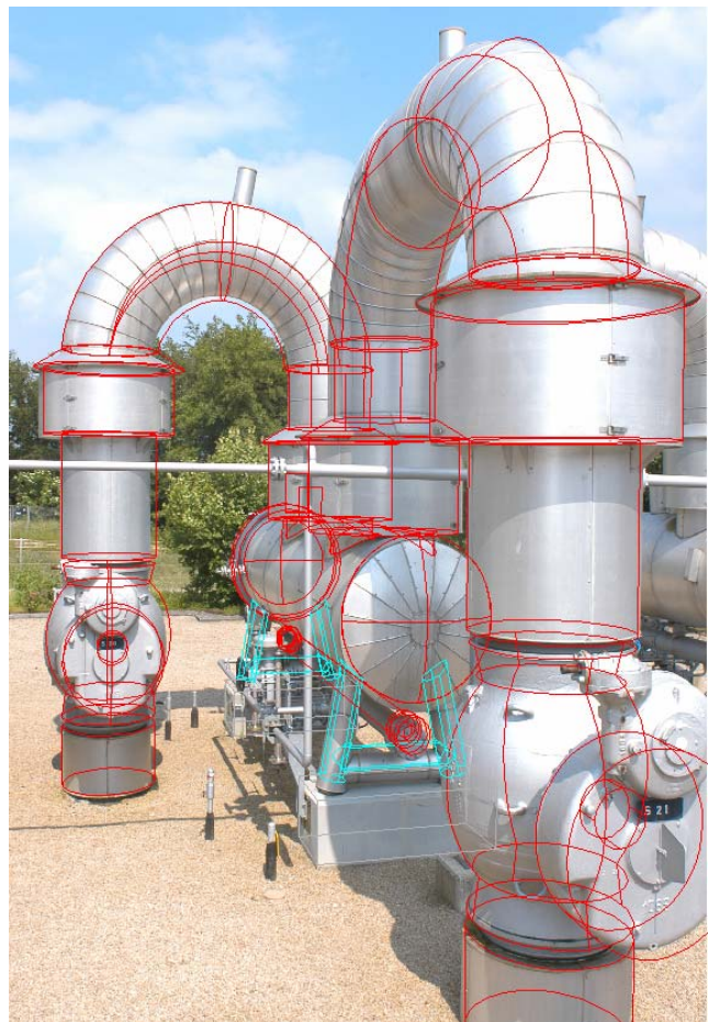
Fig. 16: Super-imposition of photograph and constructed elements
