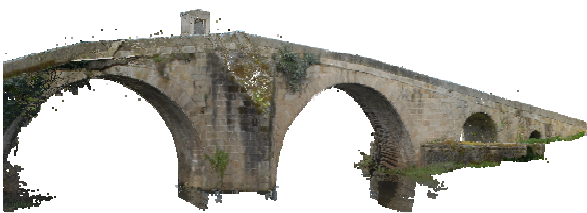
Figure 6. Coloured point cloud of Carracedo Bridge.
